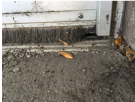
Door sweeps, like the one pictured here, go a long way toward keeping rodents out of your building. Photo credit: NYS IPM Program.
