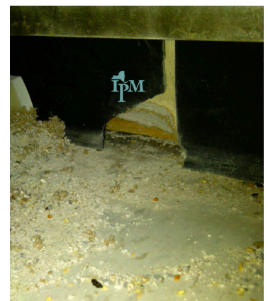
Damaged building material caused by gnawing. Photo credit: NYS IPM Program.
