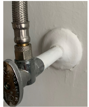
Escutcheon plates, like the one pictured here, help keep pests from entering buildings. Photo credit: Amy Hourigan
