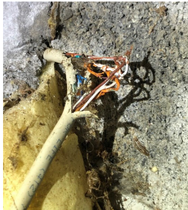
Chewed wires are a leading cause of fires. Photo credit: Susannah Krusko, MS, StopPests.org
